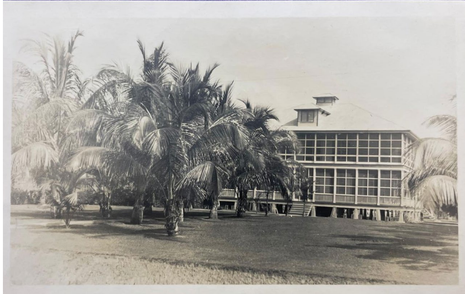
Figure 3: Image of the Cutter residence in Virginia Farm. Photograph from Rauner Special Collections Library
